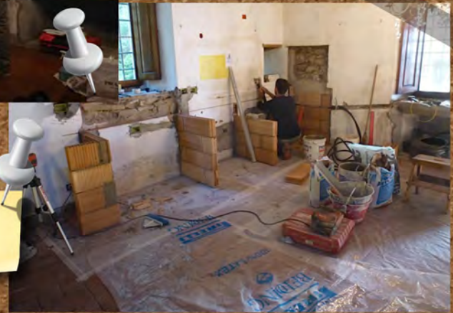
mason building supporting structure of extruded terra cotta blocks and planks
