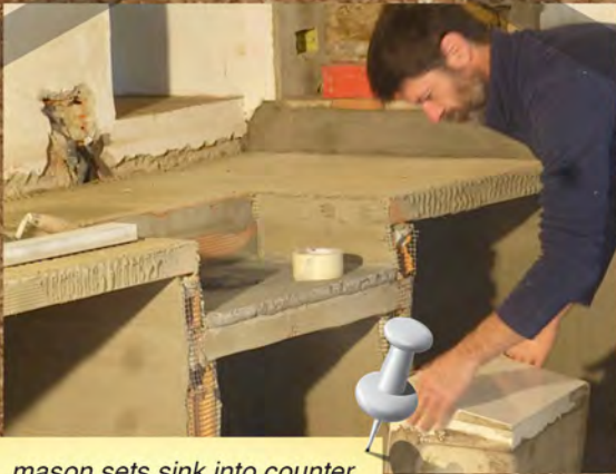
mason sets sink into counter
