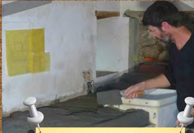
sink in place mason double coats counter, note: working drawing on yellow tracing paper taped to wall - has it been examined and approved and permit issued ?
