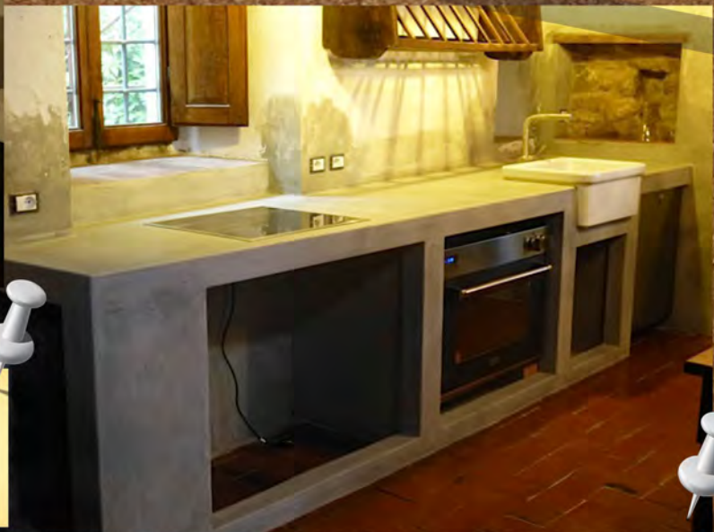
All cleaned - up, counter ready for cabinet inserts, appliances installed - electric oven and induction cook top. Walls to be painted - put that item on the punch list !
